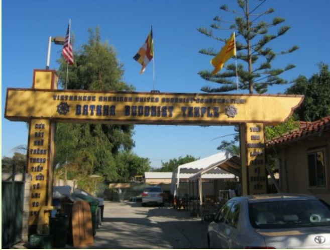
Bat Nha Buddhist Meditation Center, at 803 S. Sullivan St. in Santa Ana, is planning to replace its old buildings with a 8,551 square foot meditation center on its 1.46-acre site.
